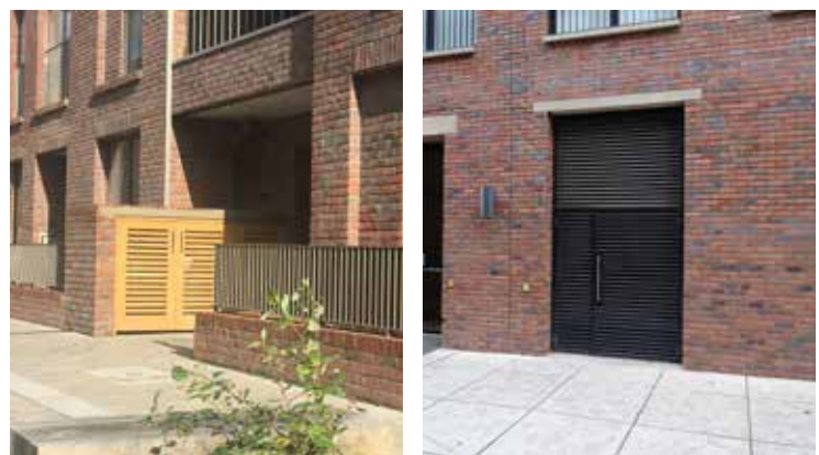
Fig 101 Examples of waste and recycling storage integrated into the overall built form of the development. Photo credits: © Allies and Morrison
