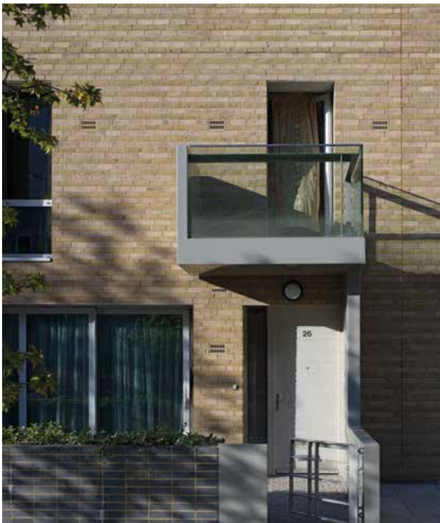
Fig 96 A direct relationship between the front of the building and the street - the front door is accessible directly from the street; windows and balconies address and add life to the street; a low boundary wall offers privacy without presenting a blank frontage
